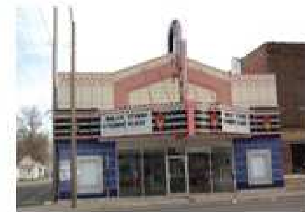
Old South Town Theater (city landmark), 1110 East South Grand Avenue
