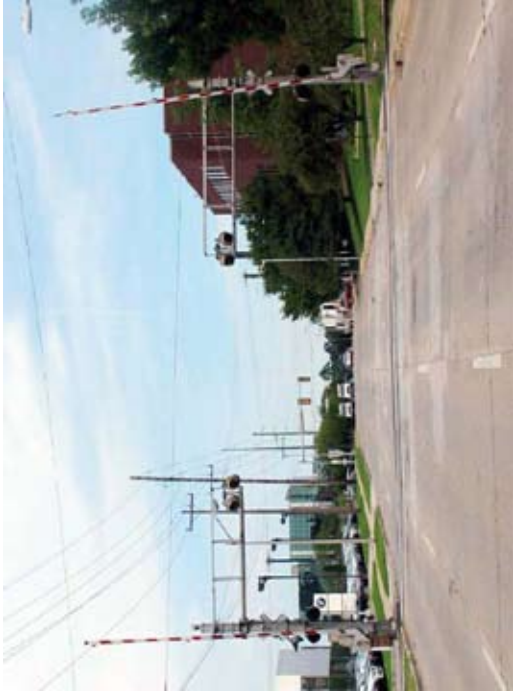
ONE - WAY STREET WITH - FULL GATE CLOSURE
