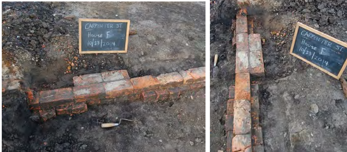
Figure 89. Details of the east foundation wall (original, front section) of House F. The double-wide brick pier and adjacent single-wide brick “curtain” wall were constructed in a single episode.
