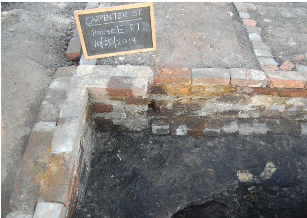
Figure 82. Two additional views of Test 1 after excavation. Top: Looking northeast. Bottom: Detail of northeast corner of foundation wall indicating presence of L-shaped double wide wall transitioning into a single course wall. The single course brick wall was laid on an initial header course which corresponded to the same width as the double-course wide wall. A similar method was also observed in the adjacent House F, and may represent a characteristic employed by Mr. Roll in his buildings.
