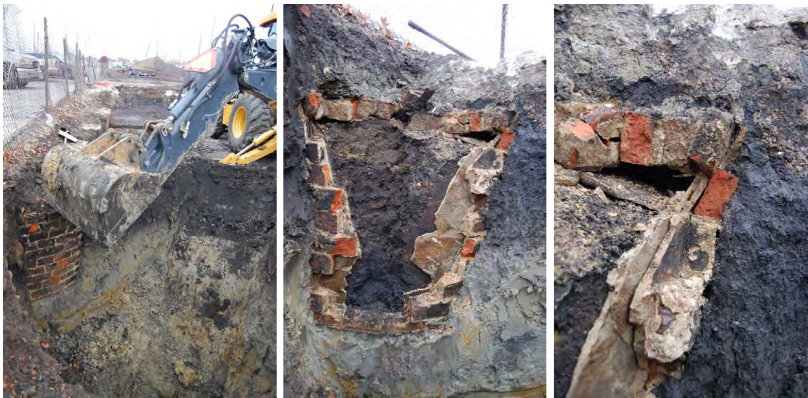
Figure 101. Three views of the cistern (House F, Feature 3) during machine excavations. Left: Beginning excavation. Middle: Cistern wall and interior contents exposed. Right: Detail of collapsed dome, displaced side wall, and multiple coats of interior mortar lining.
