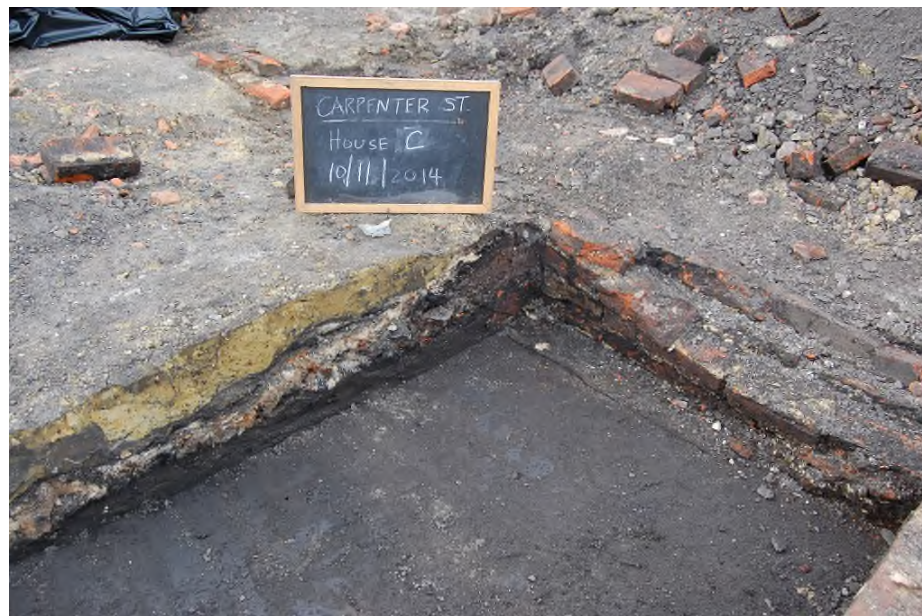
Figure 59. Two views of Test 1, House C. Left: Looking north. This test was located within the northeast corner of the rear service wing. The brick wall on the right is from the original dwelling (main house), and the deteriorated wall on the north end of the test unit is that of the rear service wing. Right: Looking northwest.
