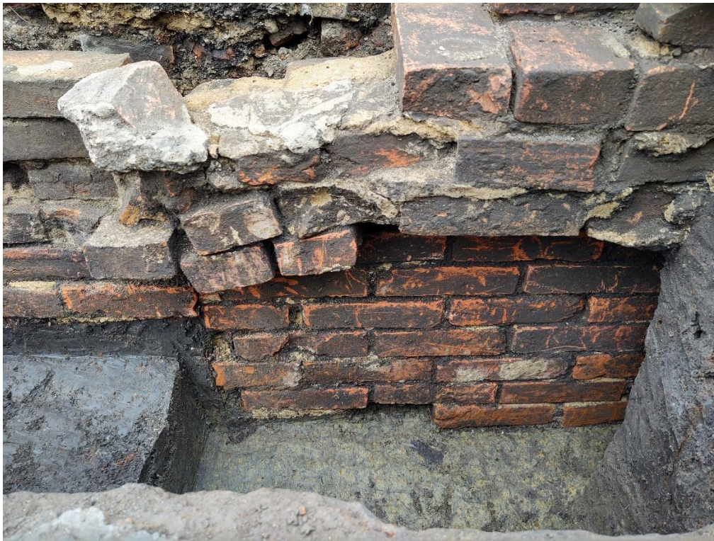
Figure 43. Top: View of the bulkhead after its interior was partially excavated and the south sidewall was fully exposed down to its base. Bottom: Detail of the bulkhead sidewall. The lower section is original and only one brick wide (Feature 16A). The upper section, which represents a later modification, is two bricks wide (Feature 16B).
