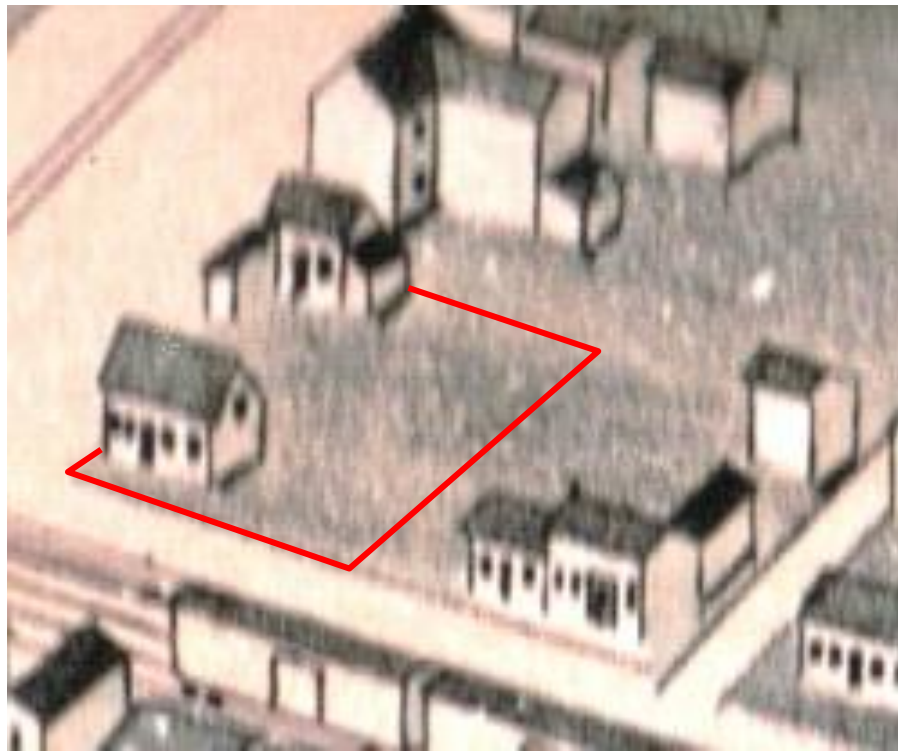
Figure 4. Top: Close-up view of Houses A, B, and C from 1867 Bird's Eye View of Springfield, Illinois (Ruger 1867), with House A lot outlined in red. Bottom: Houses A, B, and C (left to right) from the 1873 Bird's Eye View of Springfield, Illinois (Koch 1873). The 1873 bird's eye is one of the better representations of House A, in respect to door and window openings, the size of its associated lot, and the degree of separation between it and House B (located north/right of it). The suspected cabinet shop and/or barn associated with House A also is depicted by both of these bird's eye view.
