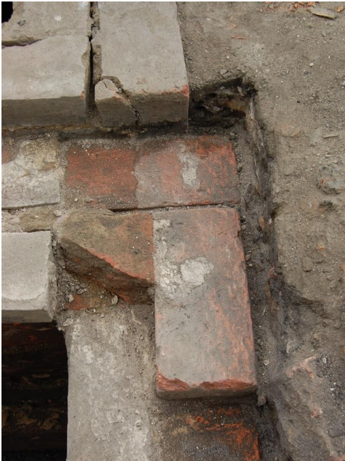
Figure 33. Top: Detail view of northeast corner of House B abutting southeast corner of House C. House B was set approximately 2-in further to the east than House C, with the two foundations not being in perfect alignment with one another. This may suggest that House C, which was frame, was laid out so that the exterior face of the framework was in line with brick wall of House B. Right: Exterior wall surface of north wall, House B, following the removal of abutting south wall of House C. This wall exhibits flush, trowel-cut mortar joints, indicating that it was constructed prior to House C. The exterior surface was not painted.
