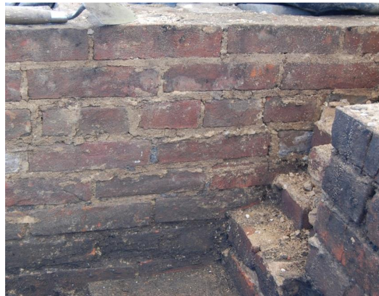
Figure 33. Top: Detail view of northeast corner of House B abutting southeast corner of House C. House B was set approximately 2-in further to the east than House C, with the two foundations not being in perfect alignment with one another. This may suggest that House C, which was frame, was laid out so that the exterior face of the framework was in line with brick wall of House B. Right: Exterior wall surface of north wall, House B, following the removal of abutting south wall of House C. This wall exhibits flush, trowel-cut mortar joints, indicating that it was constructed prior to House C. The exterior surface was not painted.
