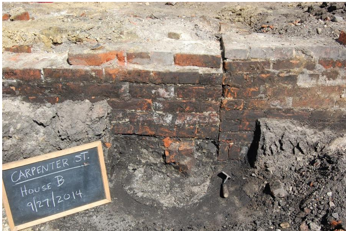
Figure 17. Top: Detail of vent opening (Feature 14) in south wall of the original house foundations. Bottom: Detail of the southwest corner of the original house, illustrating the rear service wing and the underlying post hole (Feature 6). Both views look north.
