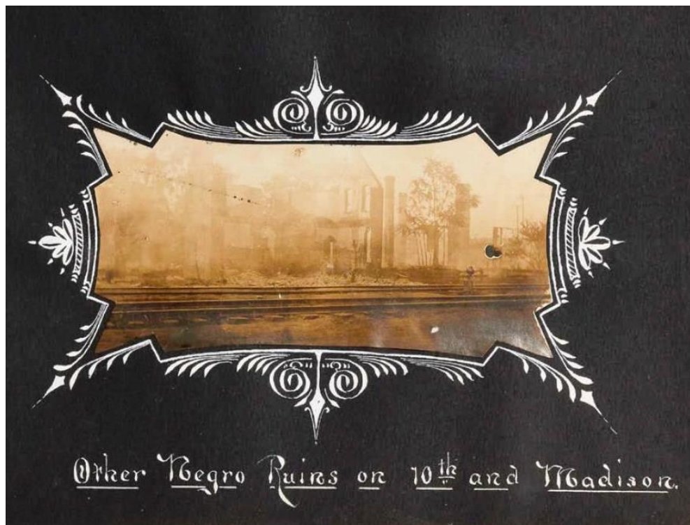
View 7f-g. Two views of the gutted two-story, brick house at 1022 East Madison Street, looking southwest. Top: Looking west/southwest with the junction of the Wabash and Illinois Central Railroads can be seen in background, with the State Capitol building in far distance ( http://library.uis.edu/archives/localhistory/riotphotos.html ; from the Booth-Grunendike Collection, Archives/Special Collections, Brookens Library, University of Illinois at Springfield). Bottom: Similar view from a 1909 scrap book (Smithsonian African American History Museum).
