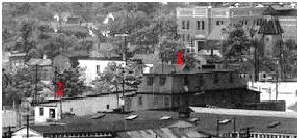
Figure 12. Two photographs taken in the mid-1930s showing developments in Wright and Brown's Subdivision (outlined in red) at that time. (Top) Aerial view, looking southwest and showing the old plaster mill on the northwest corner of Tenth and Madison (No. 1) and the narrow brick building occupied by the Ben Wright Hide Company (No. 2), which had been constructed in 1920-1. (Bottom) Another view of these buildings, looking northeast from the central business district (Sangamon Valley Collection).
