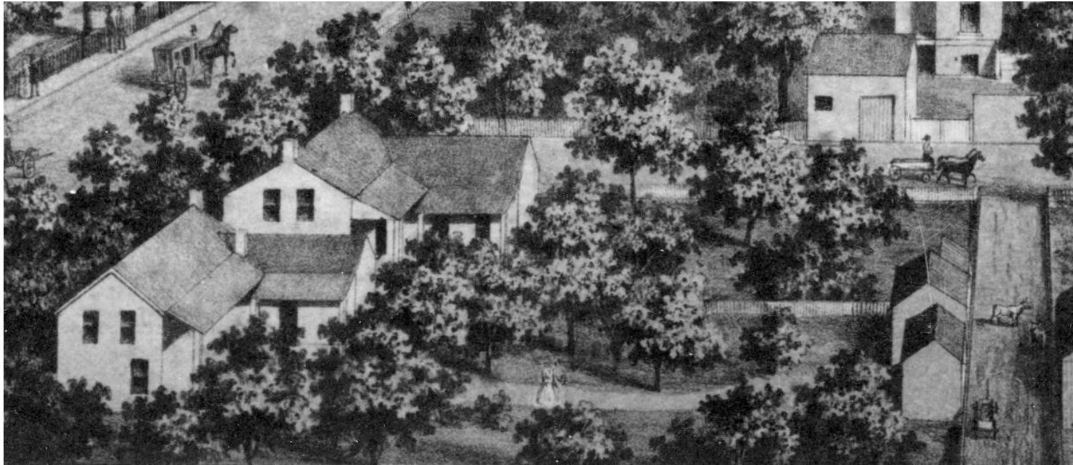
Figure 161. Detail from the bird's eye view entitled " Springfield, Illinois 1860 " (Hearting 1860) illustrating two traditional frame houses associated with two painting contractors. The northern house was owned by R. H. Zimmerman in 1854, whereas the southern house was owned by A. P. Willard. Both houses are 1-1/2 stories in height, gable-roofed, single-pile dwellings with single story rear service wings. The rear service wings are located with their roof lines perpendicular to the main body of the house, giving the dwellings a distinctive L-shaped footprint, with the kitchen wings located off the north end of the main body of the house. The placement of the kitchen wing along the north end of each cottage allows for the work porches accompanying each of the kitchen wings to take full advantage of a southern exposure. Both houses lack architectural stylistic details (such as decorative eave or return cornices). The main body of the northern house appears to be slightly wider than the southern house's main body, and the rear service wing of the northern house appears to be slightly larger than the southern house's service wing. Both houses are considered traditional I-cottages. Unfortunately, it is unclear as to the character of the front of each house, and whether they are 3-bay (one window each side of main level door) or 5-bay (two windows each side of main level door) dwellings. The northern house was constructed on two city lots, whereas the southern house was constructed on 2½ city lots. Although one house (the smaller of the two) has multiple outbuildings adjacent to the rear alley, the second house (the larger of the two, which is located on the corner lot) has no outbuildings.
