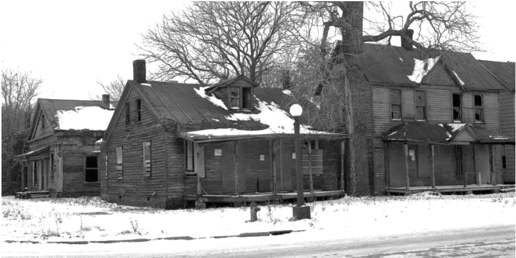
Figure 319. View of dilapidated houses located at the southwest corner Thirteenth and Adams Street, January 1965 (Mercury Studio Collections). The houses pictured are all Double-Houses (Duplexes) and represent three different historic examples of this particular house form. The 1- \frac{1}{2} -story residence at center has a similar massing as that presumed for Houses A and D. Note the double set of front entrances, and the two end-chimneys.
