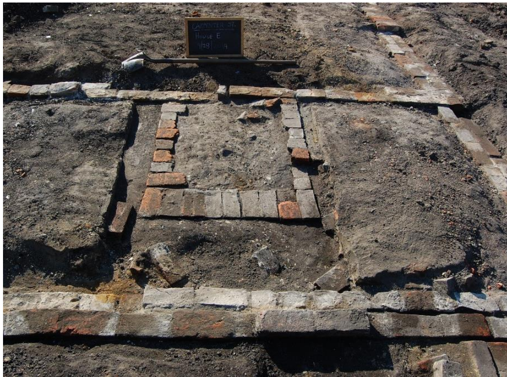
Figure 15. Two views of the original front porch stoop foundations (Feature 11) in 2014. Top: Looking east from inside house. Bottom: Looking west from outside house.
