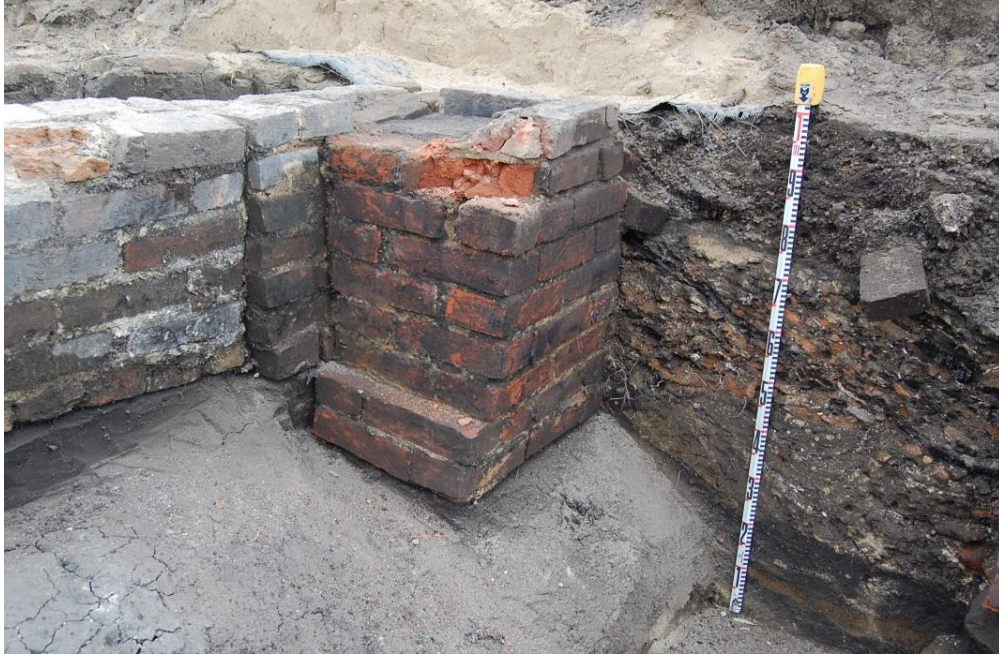
Figure 44. View of Feature 7, the brick chimney located in the southwest corner of the east room in House E. The base of the chimney cuts into the cellar fills, indicating that it was added later. The section of foundations abutting the chimney was rebuilt when the chimney was constructed (note butt joint in foundations).
