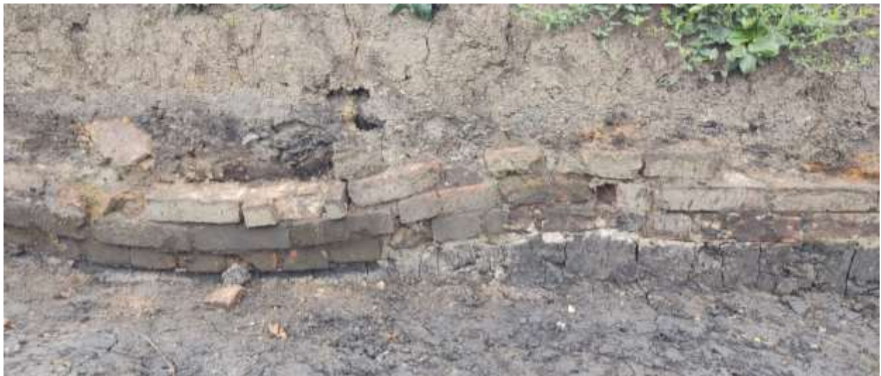
Figure 66. View of a section of the northern foundation wall of the original house, illustrating significant settling that had occurred along this section of the perimeter foundations. The boggy character of the soil in this area may have contributed to the subsidence in the foundations.
