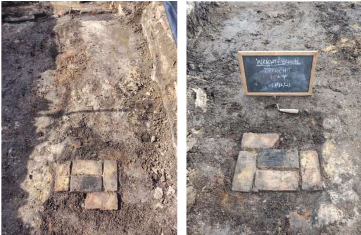
Figure 34. Phase II investigations at Price-Edwards Site, showing brick pier associated with rear service wing (Feature 4). Left: View looking west, with eastern wall of house foundations (Feature 1) visible in background at top of image. Right: Detail of pier (Feature 4) looking east.
