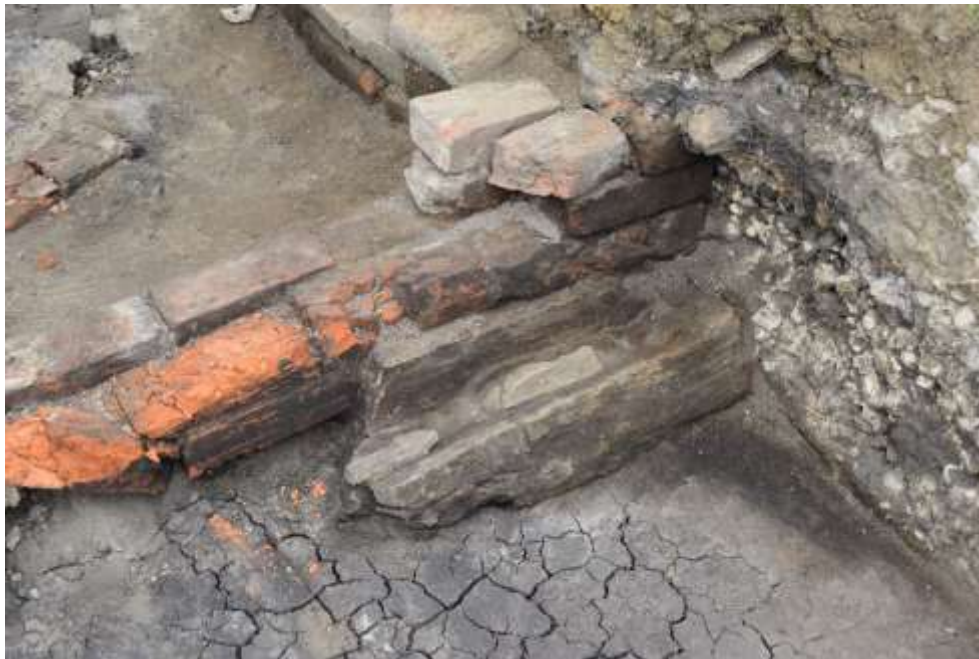
Figure 63. View of the northeast corner of the original house, showing sandstone pier over which brick foundations have been laid. This pier is discussed as Feature 29C.
