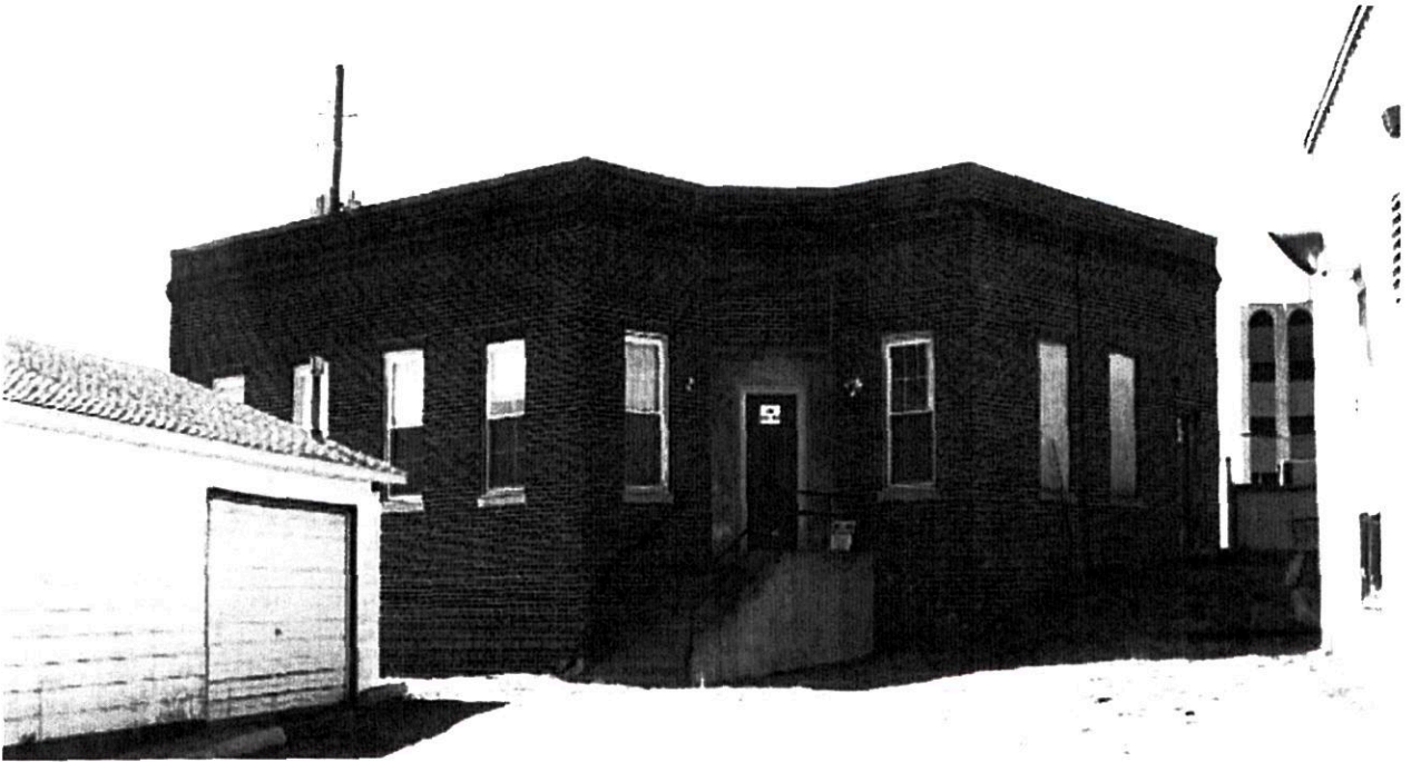
Peabody Coal Company Office, 2135 South 9th Street
