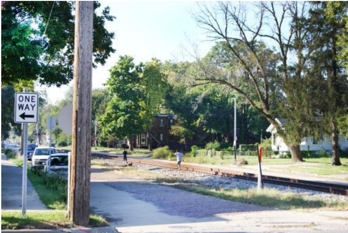
Exhibit 2-3. Existing Tracks on 3 rd Street
